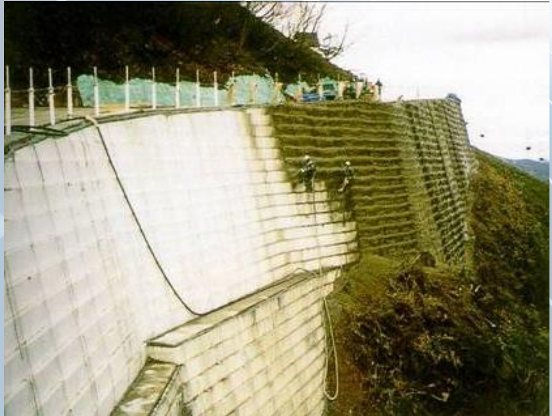
Hillside Restoration in Japan
